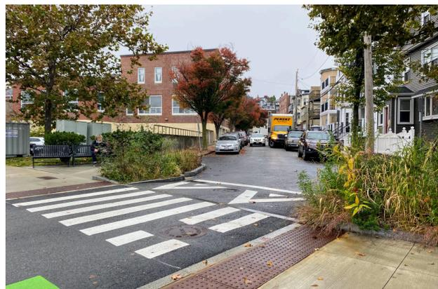
*Pictured:* Example of traffic-calming green infrastructure curb extensions with vegetation on both sides of a crosswalk in Somerville, MA.
